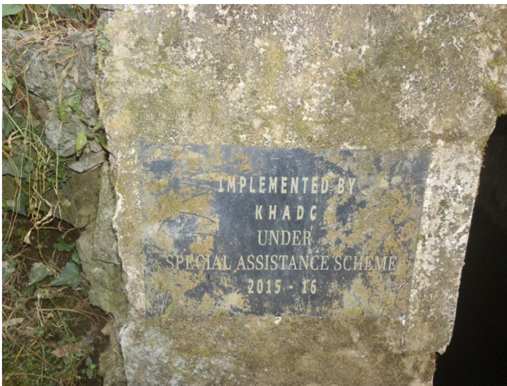
Fig. 25: The plaque of the KHADC-funded project
