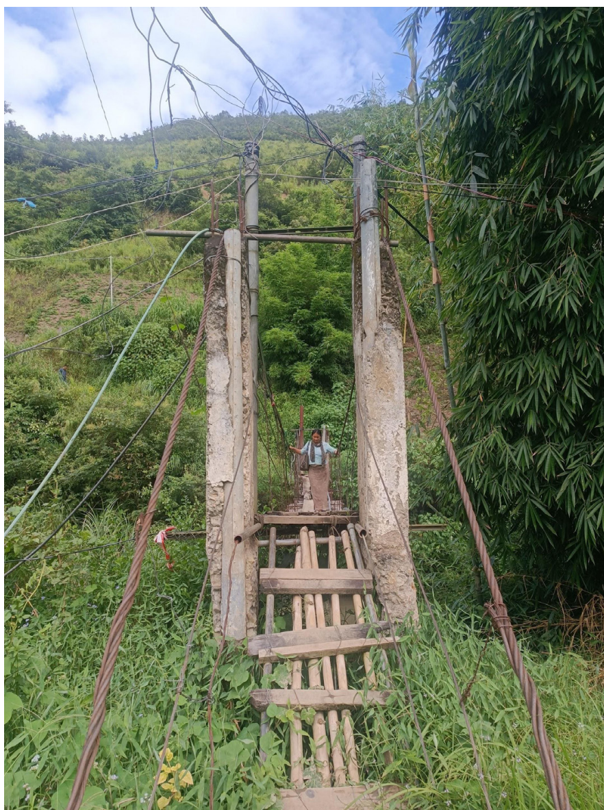
The wooden bridge that leads to Seinai's house, Senapati district, Manipur. Photo: Schulu Duo, 2023.
